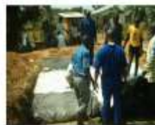
c) Closing the silage by wrapping and fixing the plastic sheets
