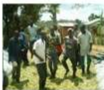
b) Filling the pit with material and compressing it for removing air
