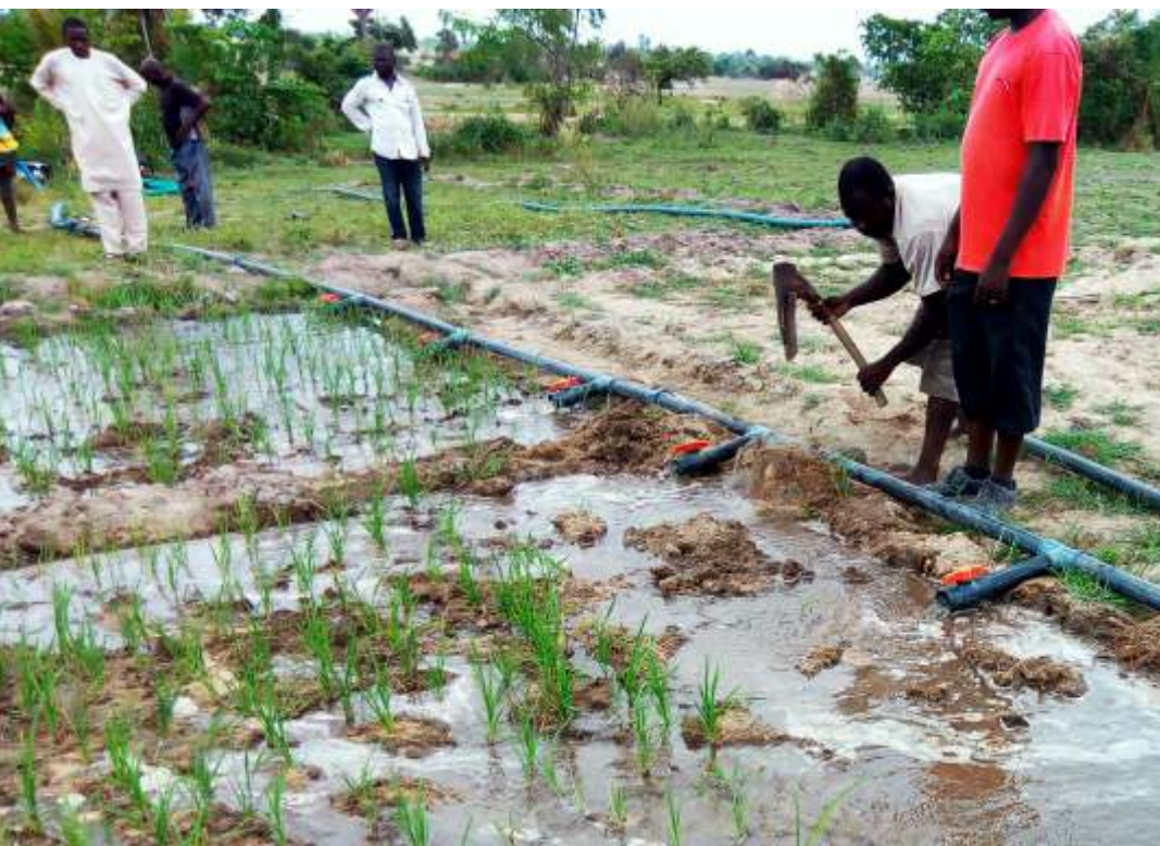
Laying the pressurized PVC pipe distribution system in Nasarawa
