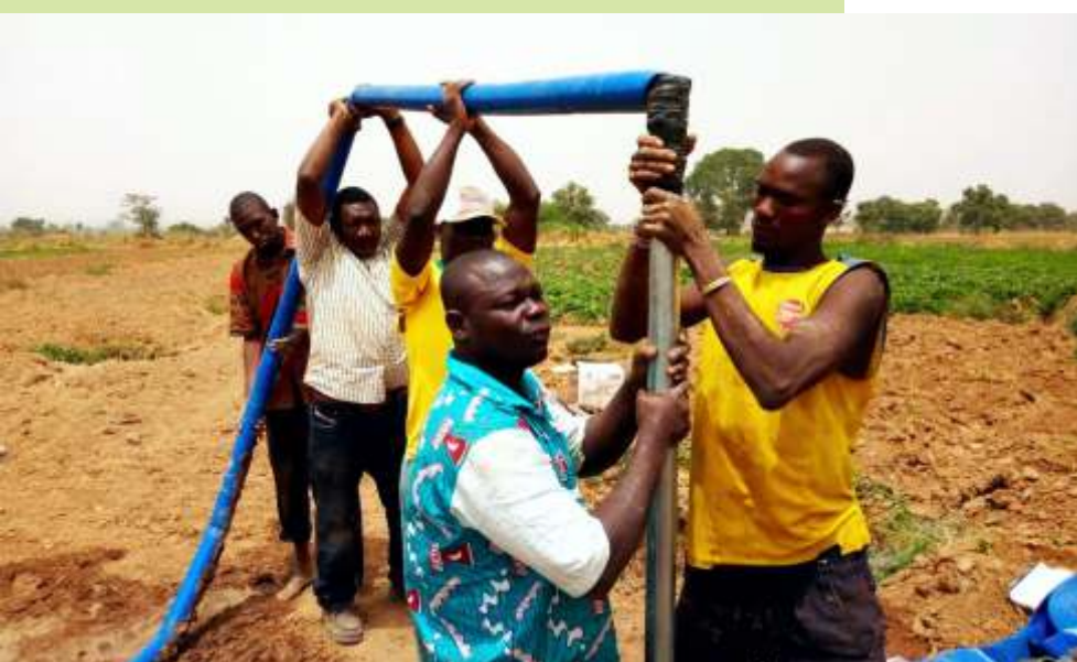
Rice farmers in Sikasso, Mali participate in the installation of tube wells
