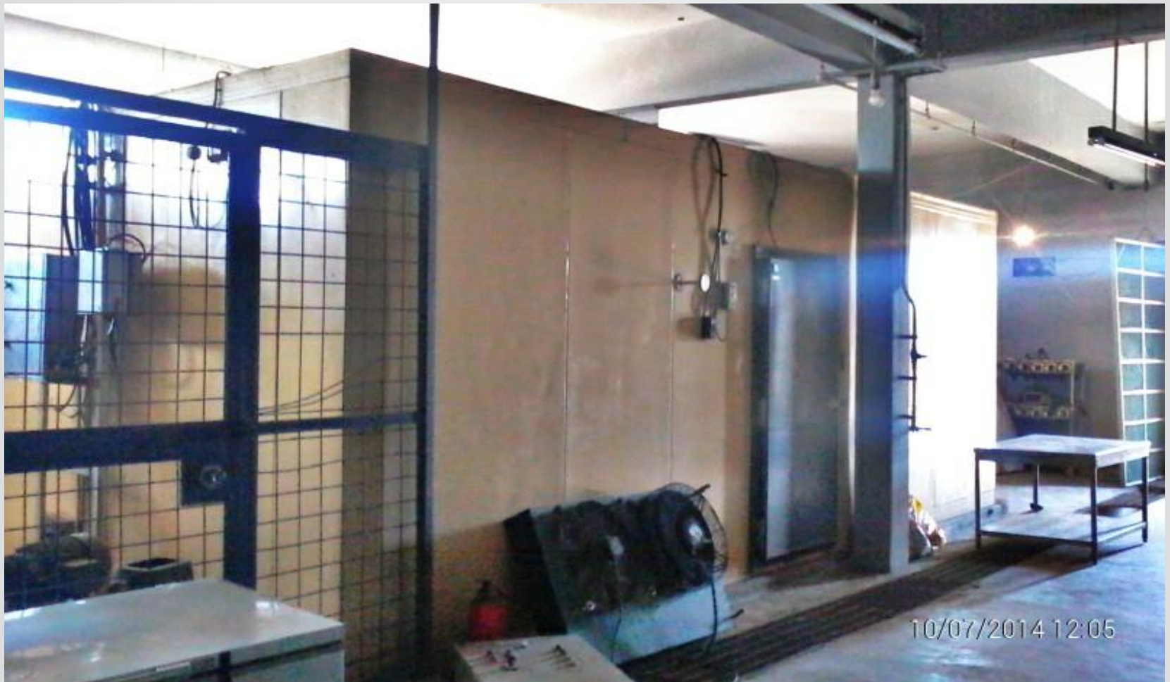
Plate 4: NIOMR Cold Room Facility
