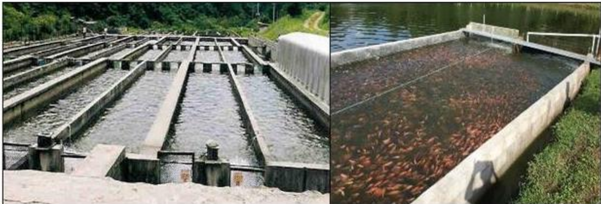
A network of parallel raceways (left) and red tilapia in an intensively managed raceway (right, credit: Global Seafood Alliance)
