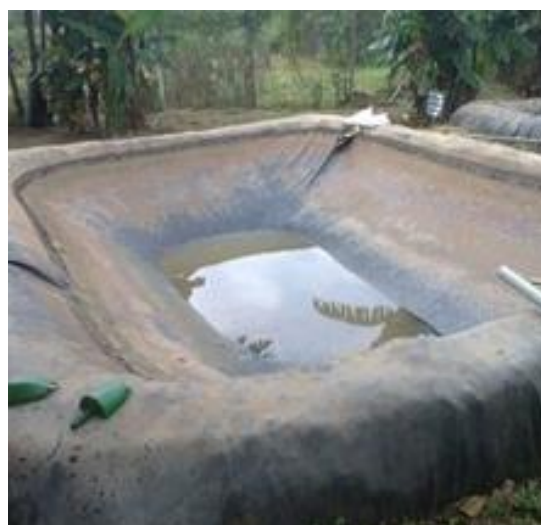
Excavated pond with liner
