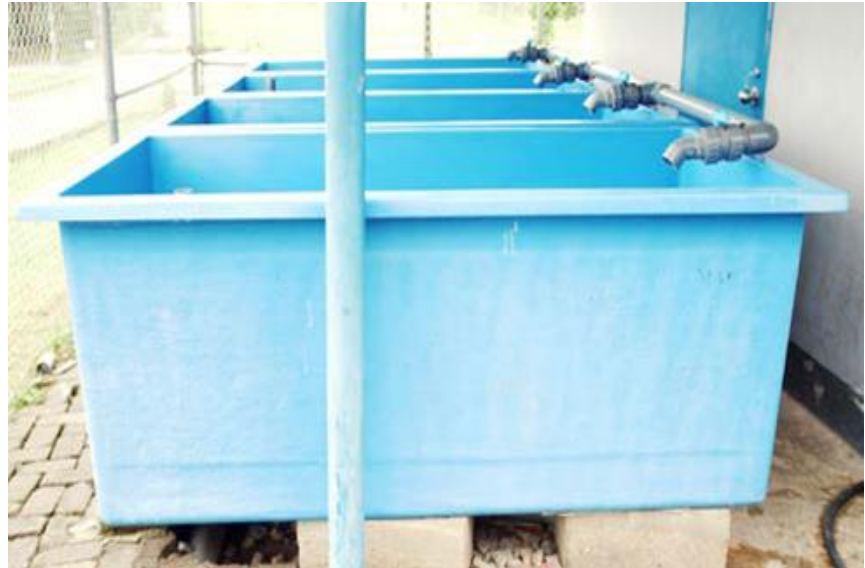
Flow-through tanks with single use of water
